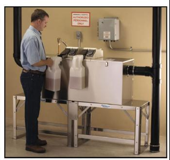
pretreat kitchen waste water flows of 25, 75 and 125 gallons per minute. The W-250-AST treats point source kitchen flows like those found in fast food restaurants and small-flow facilities. The W-750-AST and W-1250-AST Grease Removal Units are geared towards larger facilities like hospitals or casinos, where grease removal from multiple kitchen drain points is important.
